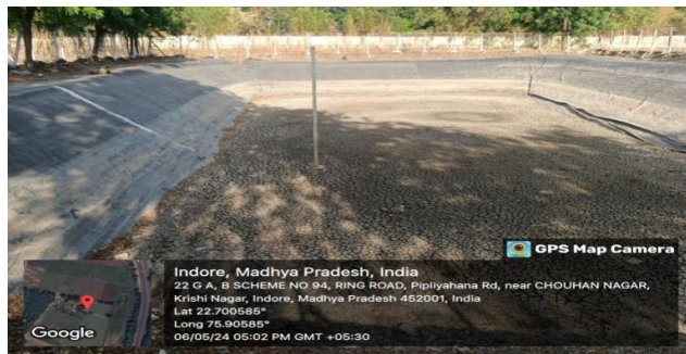
Rain water percolation & Harvesting tank at (dryland percolation tank)
