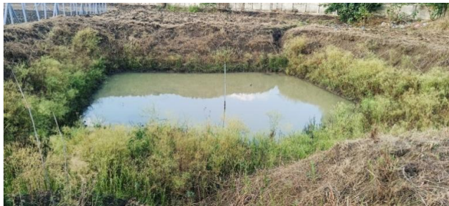
Rain water percolation & Harvesting tank at (dryland percolation tank)
