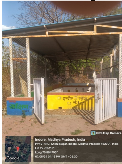
Solid waste management pit provided by IMC Indore at girls hostel building
