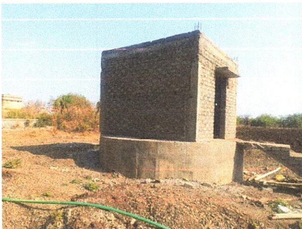
Establishment of sump well for water storage
